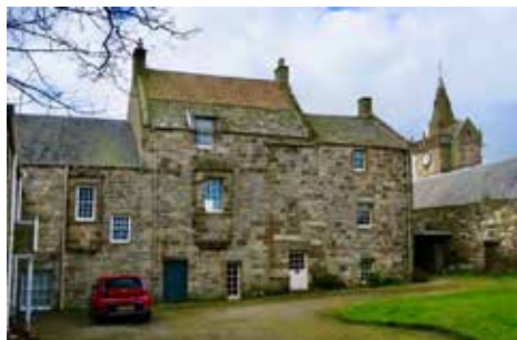
Great House from courtyard
